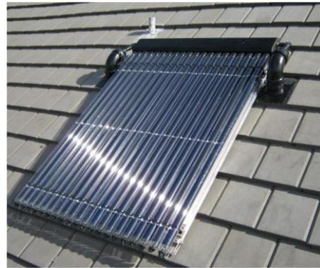
Solar thermal collectors (panels) on a roof, shade structure or other location absorb solar energy and the Solar fluid circulated through the collectors by a low-energy pump delivers heat to a water storage tank. When users need hot water, the solar-heated water in the storage tank pre-feeds the primary water-heating system.
