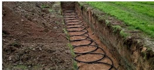
**Horizontal Ground Loop.** The simplest option; with the pipe buried at 1m, laid straight or in a 'slinky' coil to reduce the length of the trench.
